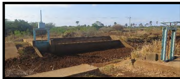
Image 30: Main canal with secondary off-takes/gates, note the amount of settled sediments
