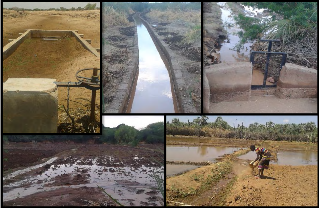
Image 17: Images of different Spate irrigation projects using structures to take water from wadi's towards the fields
