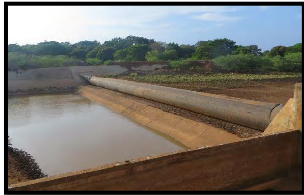
Image 29: Rubber dam when inflated
